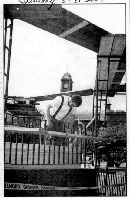
Brian Gallien of Ironwood Restoration in Marlow, N.H., works on the bandstand at Broad Street Park in Claremont. The structure was damaged in a storm last spring and repairs are expected to take a couple of months. (Wayne Carter photo)
